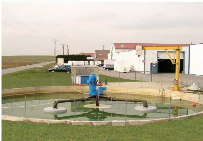
Concrete test tank - Volume 1000 m 3
