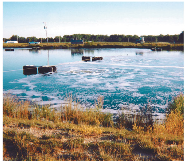
The AIRE-O 2 ® 275 aerator is pictured above mounted in a dual pontoon assembly. In the "bubble" product photo, the unifloat option is shown.
