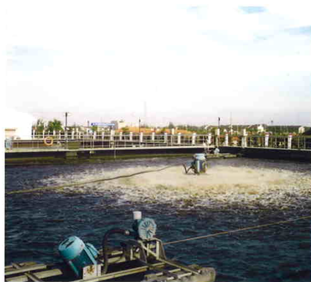
The energy-efficient AIRE-O 2 TRITON® process aerator's dual mode feature combined with the AIRE-O 2 TURBO®s.
