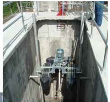
Triton aerator/mixer on slide rail system is easy to install and maintain.
