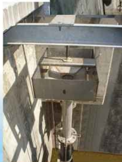
The Wagner Fluid Systems four-sided controlled decanter insures a high quality effluent.
