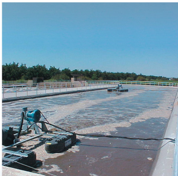
The Aire-O 2 Triton® aerator/mixer, the heart of the Tri-Oval® System, integrates fine bubble aeration with a low speed mixer capable of providing complete mixing to 33 feet (10m) deep.
